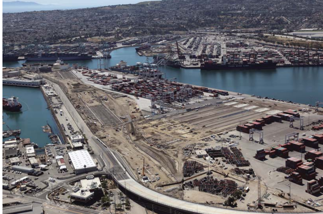
Griffith Company is building the $106 million Berth 142/143 Backland Improvement Project at the Port of Los Angeles.
