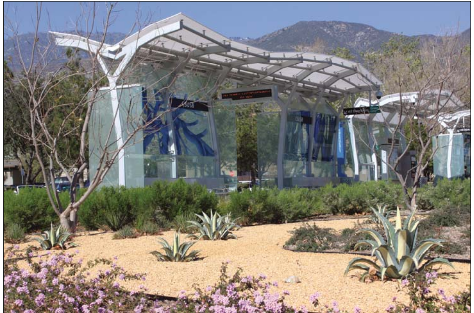
Griffith constructed the $80 million sbX E Street Corridor Project in San Bernardino.
