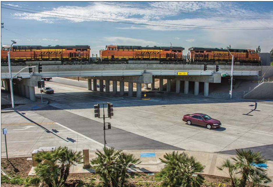
The $24 million Valley View Grade Separation project in the City of Santa Fe Springs was another recent Griffith job.
