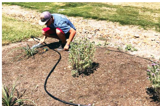
Each plot is individually irrigated. Drip irrigation is being installed here.
