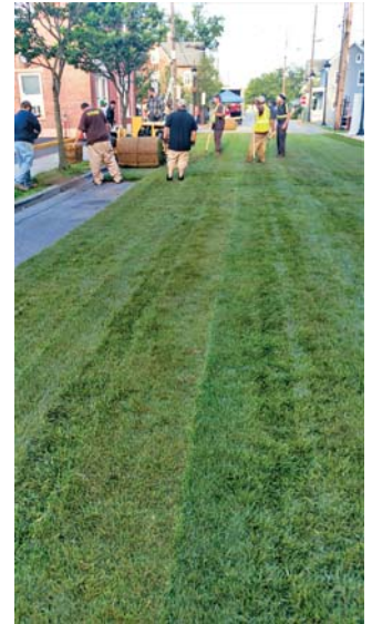
The street is almost ready for a day of fun on natural grass. Photo courtesy of John Coombs, Sr.
